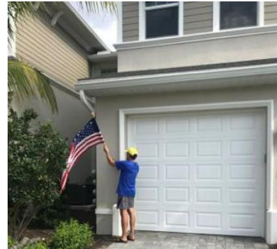
Garage wall facing the street opposite of the lamp and unit number plaque
