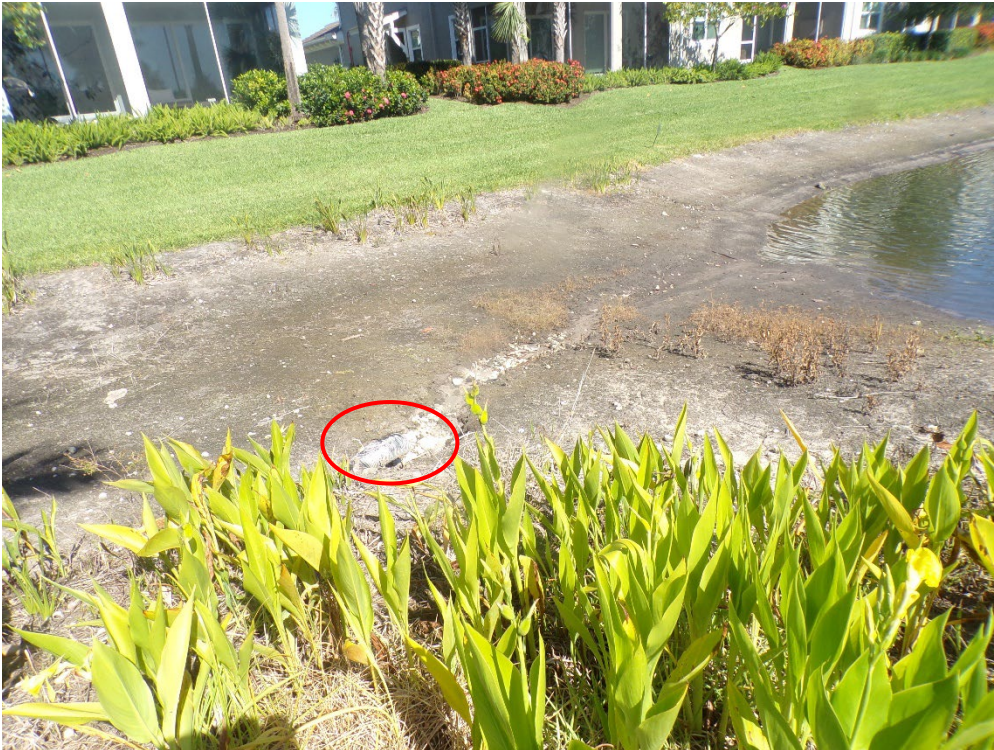
View of exposed pipe.
