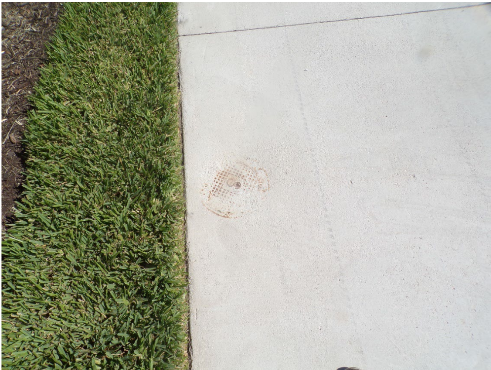
View of inaccessible drain cover.
