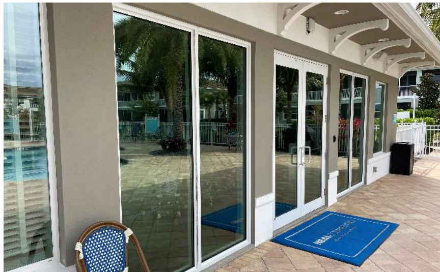
Photo 2.3.3-1: Windows and doors appeared to be properly caulked
