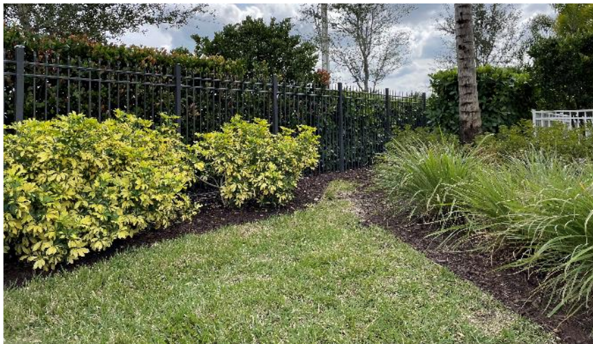
Photo 2.1.2-2: Typical section of perimeter fence
