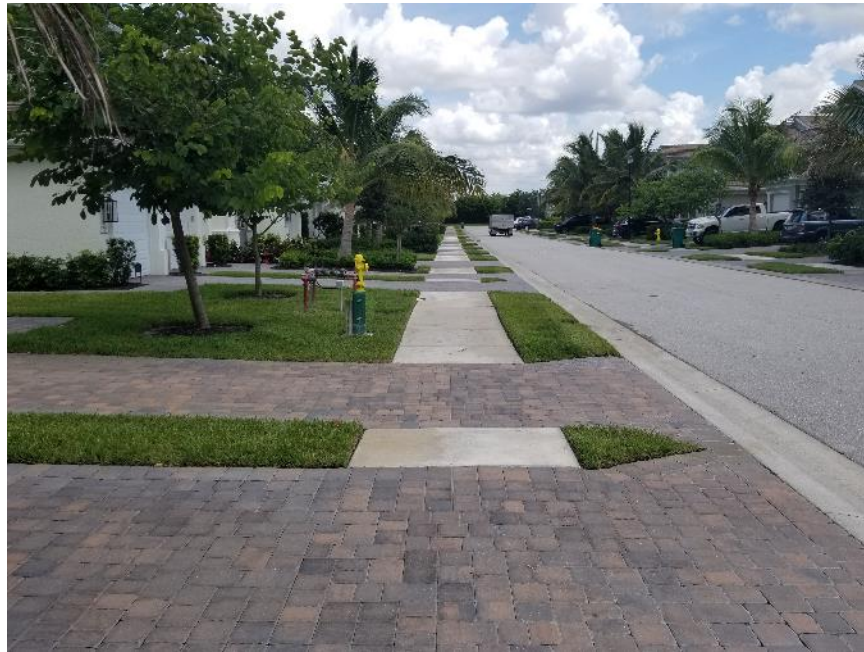
Photo 2.5.3-2: Typical view of sidewalk
