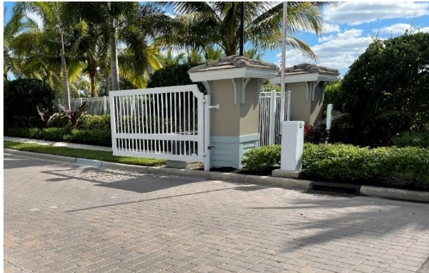
Photo 2.2-4: General view of barrier arm and swing gate
