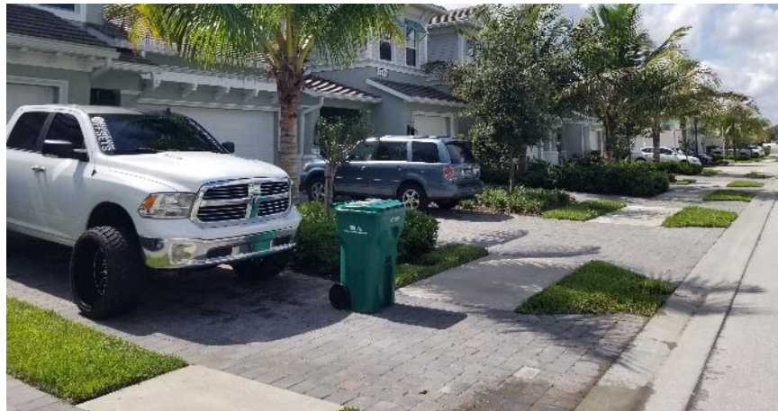
Photo 2.5.3-1: Typical view of sidewalk
