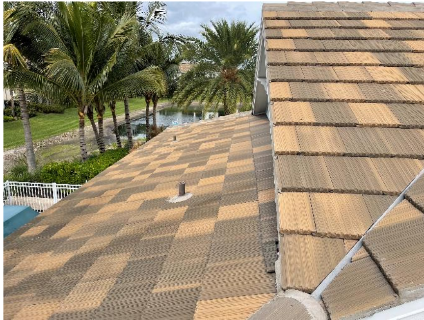
Photo 2.3.2-1: General view of clubhouse roof
