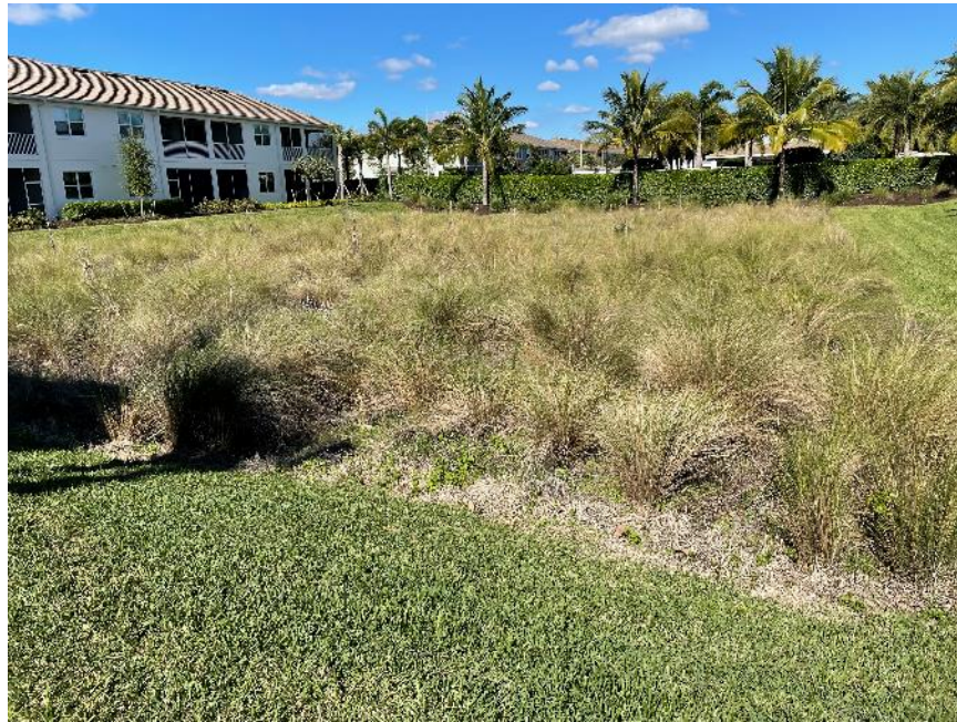
Photo 2.7-2: General view of dry detention area
