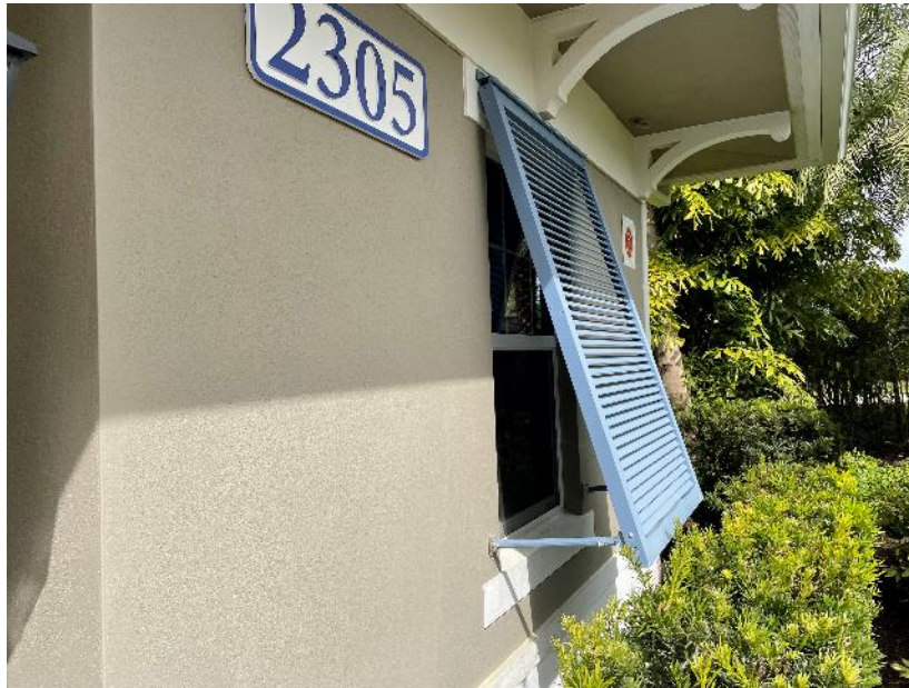
Photo 2.3.4-1: Typical clubhouse exterior paint condition
