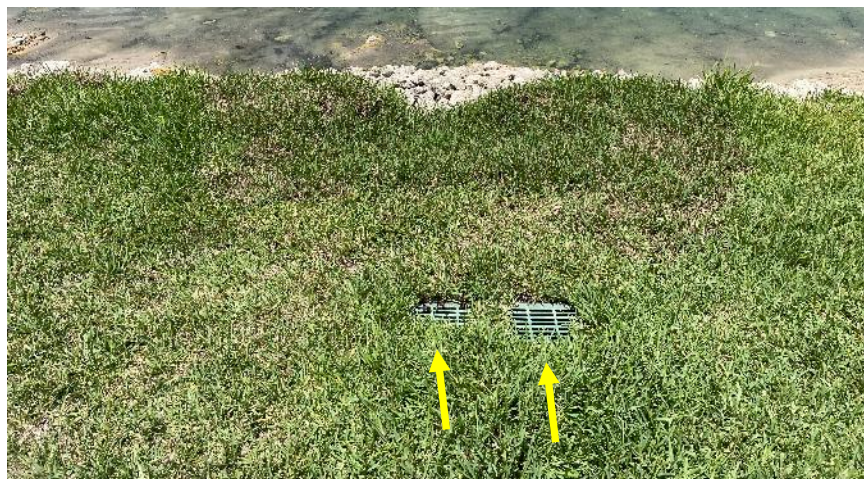
Photo 2.7-6: Drainage structures adjacent to erosion at south side of Lake 2B
