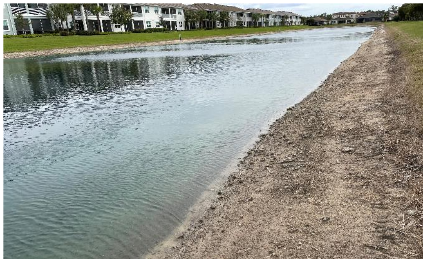
Photo 2.7-3: General view of Existing Pond – Lake 2C
