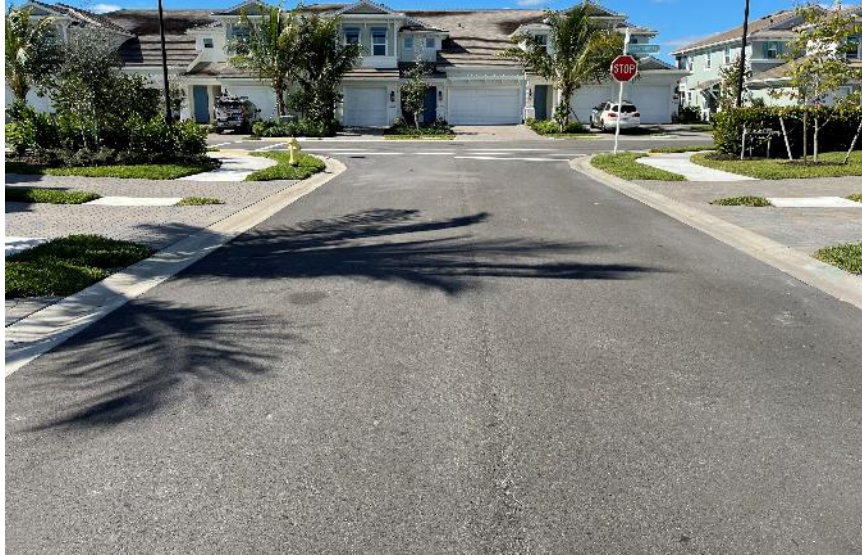
Photo 2.5.1-1: General view asphalt pavement on Priory Lane
