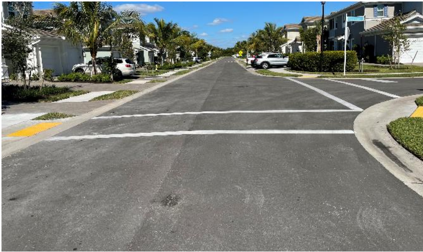
Photo 2.5.1-4: General view asphalt pavement on Sawyers Hill Road
