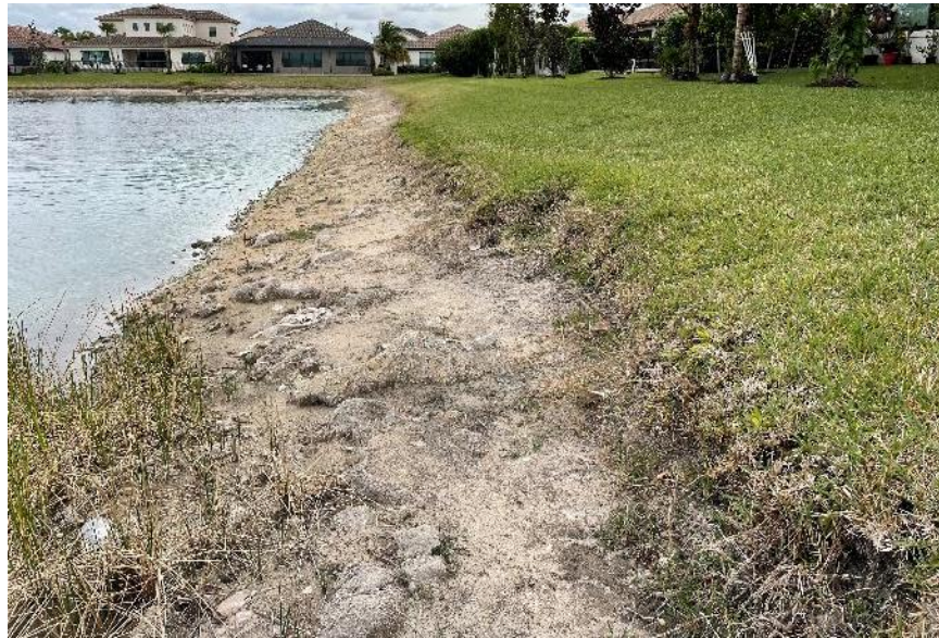
Photo 2.7-4: Isolated erosion at west side of Lake 2B
